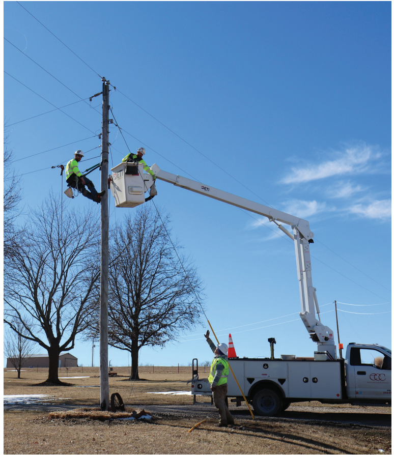
Contractors string some of the first strand wire for fiber.
