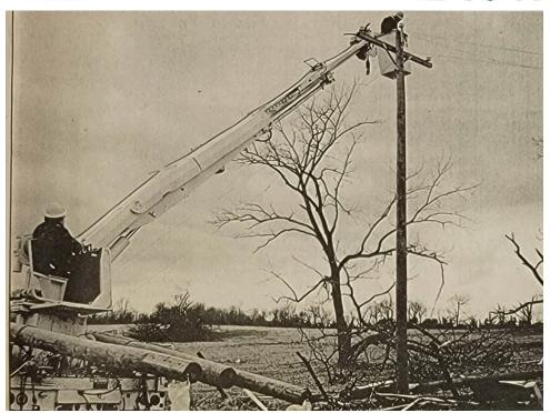
Pictured to the left is Linemen with Sac Osage Electric working to restore power in March of 2006 after a strong F2 tornado traveled from Virgil City through the BlackJack
