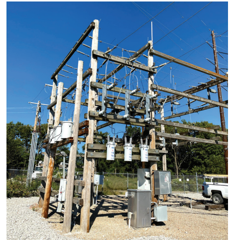
The old Tabervillie substation was a wooden structure designed to be temporary. It served the cooperative for many years.
