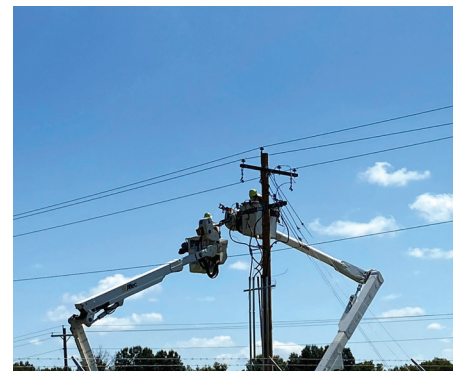
Linemen, Dustin Bray and Jared Asmus, worked high in buckets to complete the cut-over from the mobile sub to the new Tabervillie substation.
