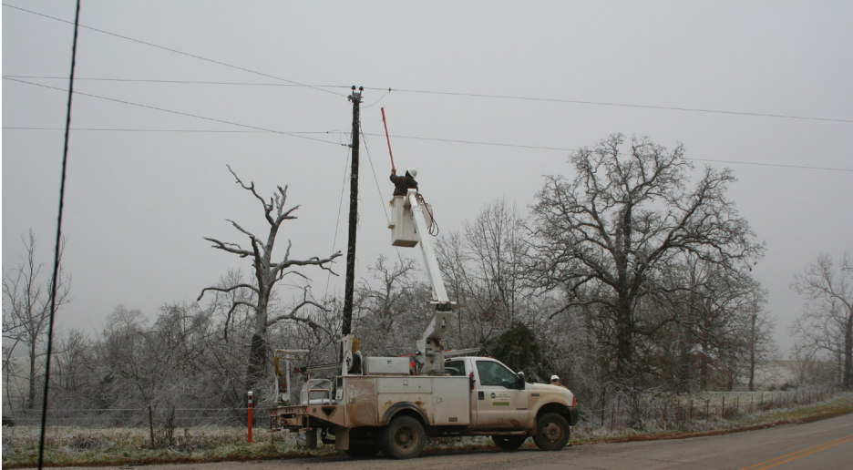
Linemen, Kent Henry and Brian Fugate, restore power during an ice storm in 2007.
