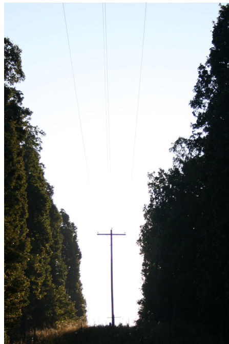
A properly maintained right of way as pictured above will reduce costly and inconvenient outages.
