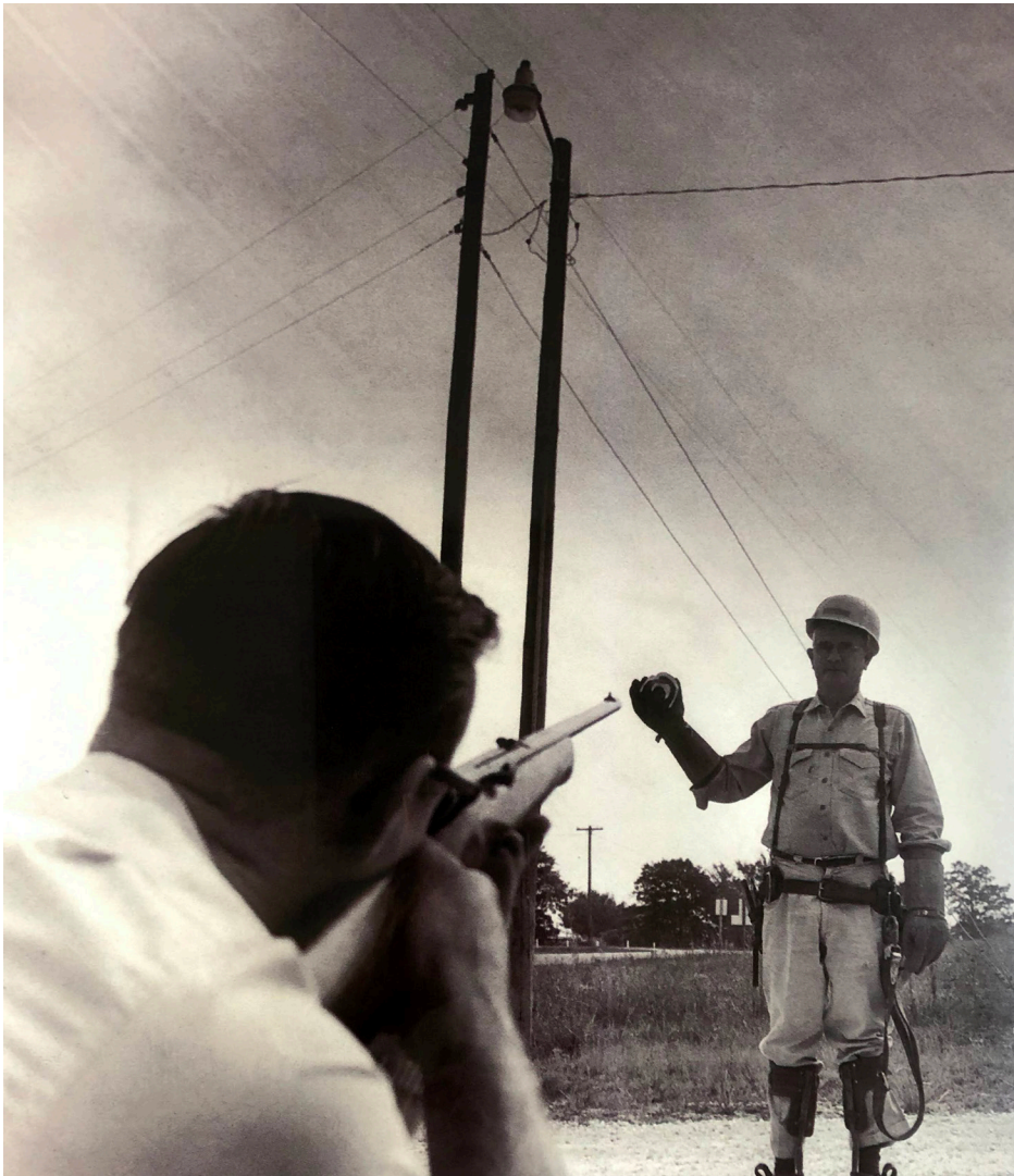
In this 1967 photo Line Superintendent, Ray Fortney holds a cracked insulator as Member Services Advisor, Walt Ryan, aims his rifle to illustrate the cause of many service outages.
