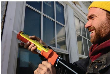
Before applying new caulk, clean and remove any old caulk or paint with a putty knife, screwdriver, brush or solvent. The area should be dry before you apply the new caulk.
