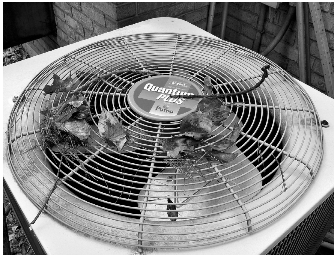
Adequate air flow is key to your air conditioner's efficient operation, so keep your unit free of leaves and other debris.
