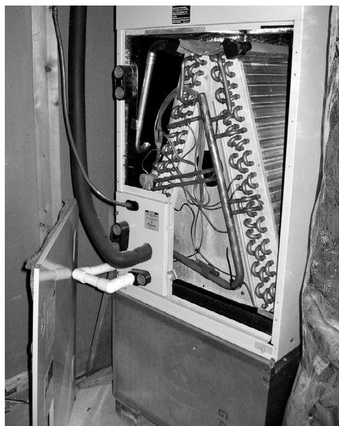
Cleaning the evaporator coils inside your indoor air handler unit will improve the unit's efficiency.
