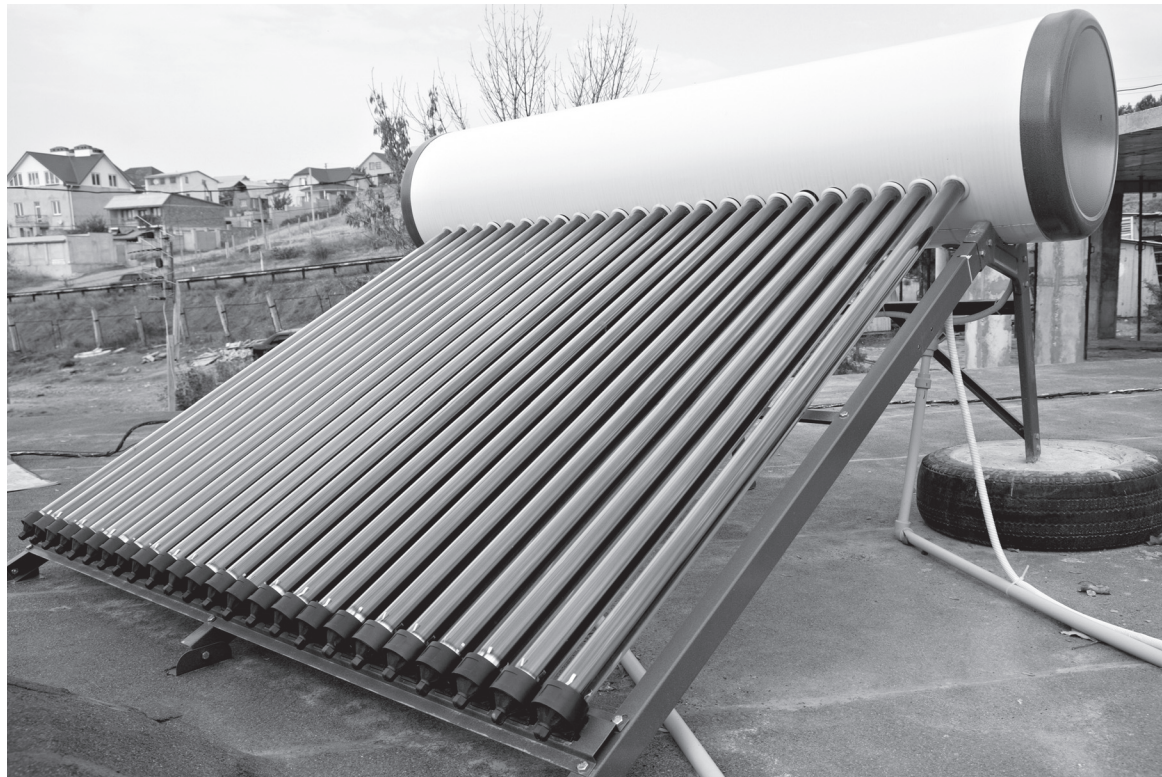
Whether you invest in a complex vacuum solar water heating system, such as seen above, or a simple, do-it-yourself kit, do your homework and learn about solar water heating and the energy savings that can be achieved.
