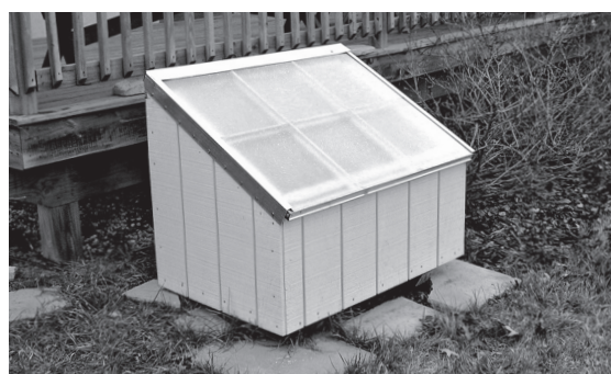
This do-it-yourself solar water heating kit uses a batch design to preheat incoming cold water.
