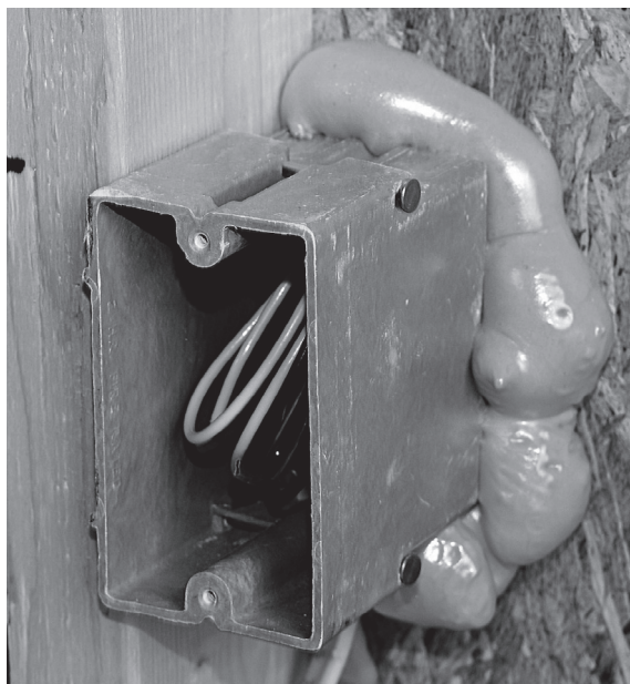
Above: Caulk gaps between window frames and rough wall openings to seal your home's exterior thermal envelope and improve energy efficiency. Below: Spray expanding foam behind conduit boxes to seal openings where electrical wires pass through outside walls.
