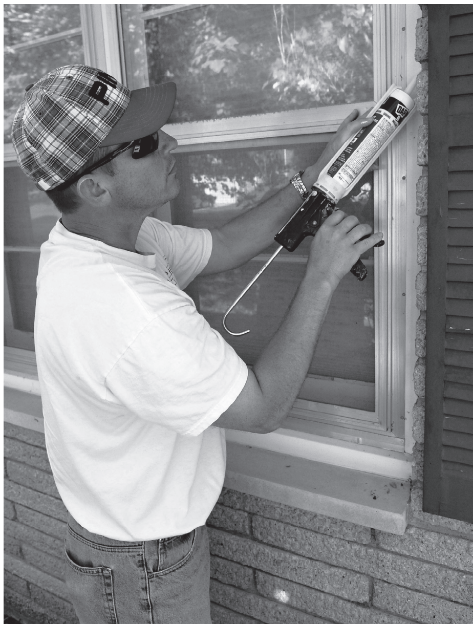
Above: Caulk gaps between window frames and rough wall openings to seal your home's exterior thermal envelope and improve energy efficiency. Below: Spray expanding foam behind conduit boxes to seal openings where electrical wires pass through outside walls.
