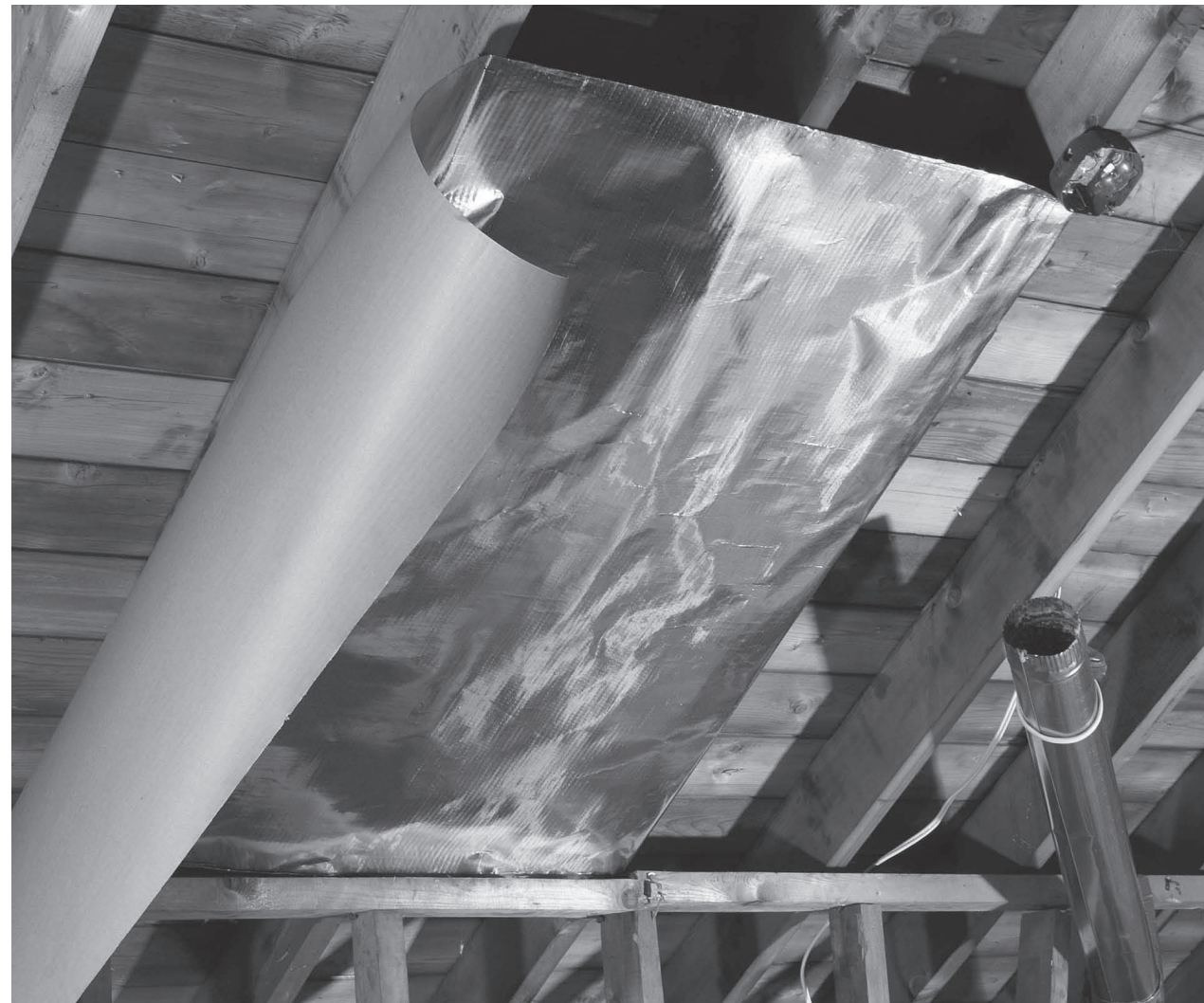
A construction stapler, utility knife and a long straight edge are really all you need for this do-it-yourself job.
