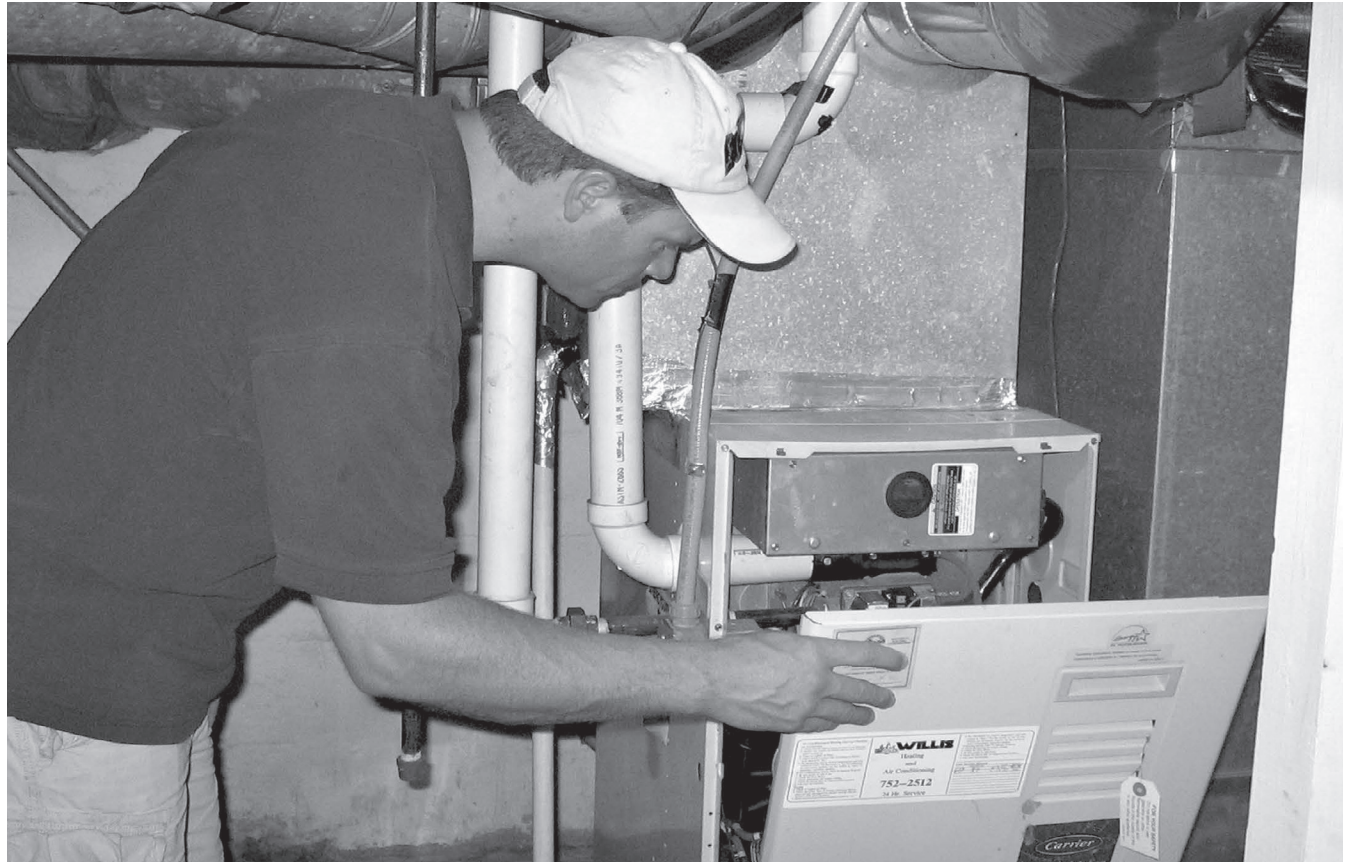
Before doing anything, turn off the electric circuit breaker to your furnace before beginning your tuneup. Remove the cover from the burner and control portion of a condensing gas furnace to inspect.
