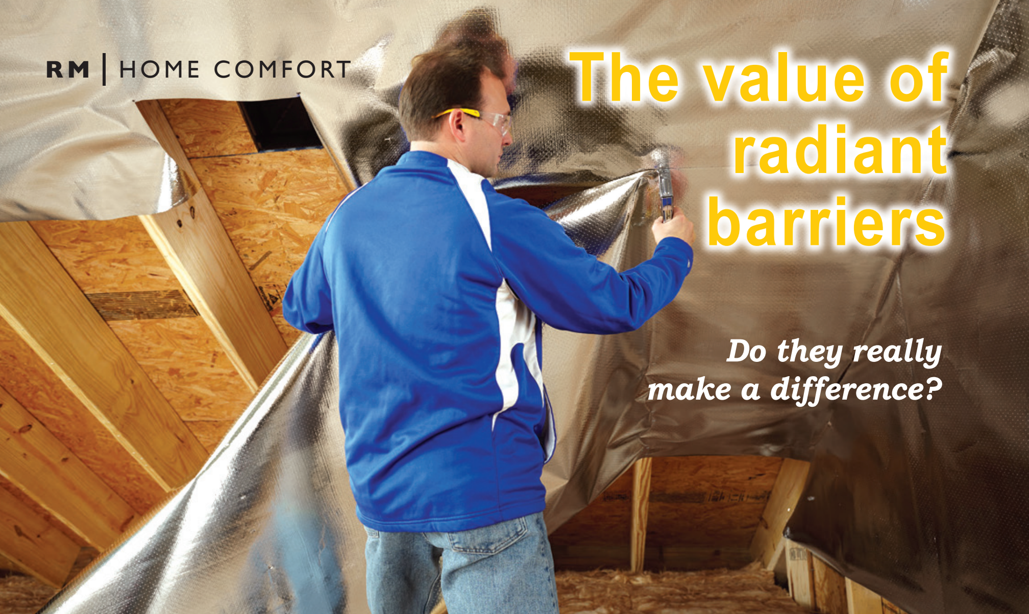
Aluminum foil is placed under the framing supporting the roof, reflecting unwanted radiant heat upward and out of the home. Photo courtesy of Reflective Insulation Manufacturers Association International.
